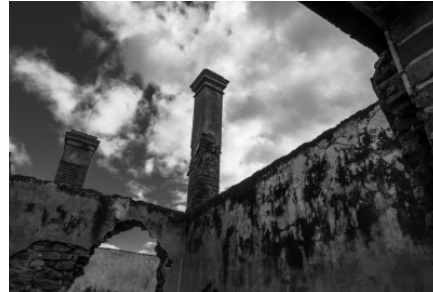
Old Station House Acceptance David Barrett
